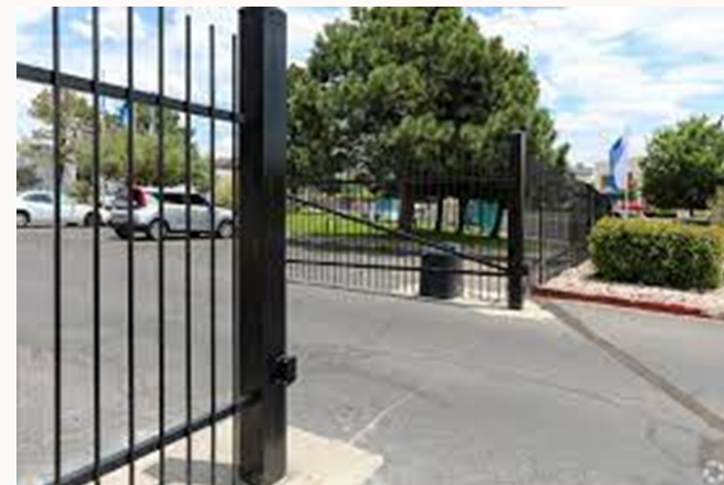
The Arioso apartments had a major improvement for calls for service due to crime prevention standards being implemented. A large part was due to installing automatic gates and fencing.
